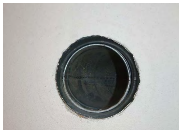
Abbildung 202: WNG ID 820: ABL-Rohr, Bad
