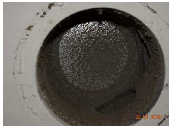
Abbildung 170: WNG ID 730: ABL-Rohr, Bad
